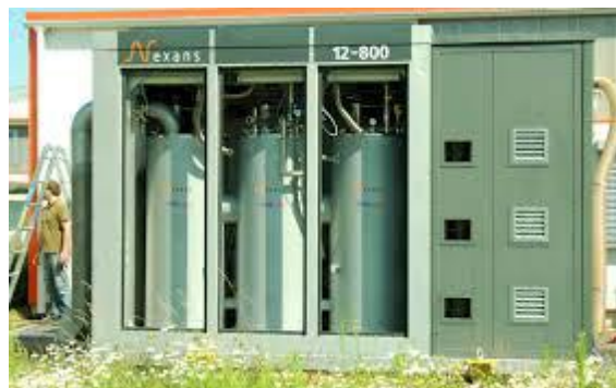
Fig.2. Superconducting FCL
